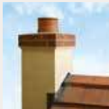
Brick or Stone Chimney (Class 1)
