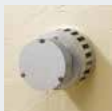
Balanced Flue (No chimney required)
